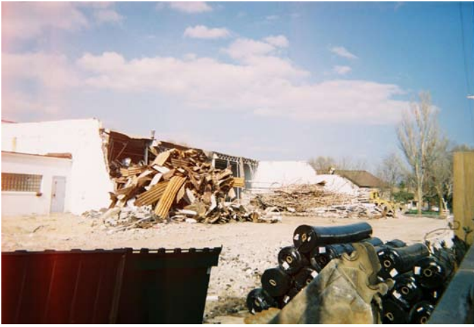
Demolition activity at the Cedar Creek Plant 2 site
